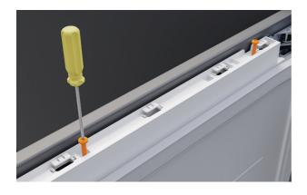
1. Fit the top cover using two supplied Phillips screws. Ensure the flat side faces away from the panel.
