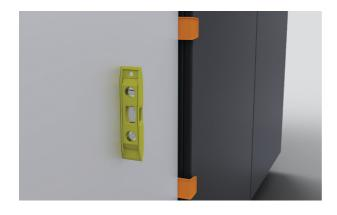
**4.** Ensure all depth gauges are flush to the front of the alcove and front of door is level.
