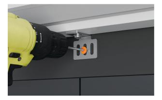
**2.** Fit an additional screw through the bracket to lock panel into position.
