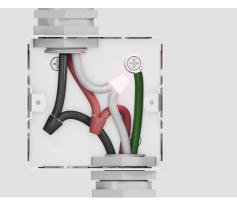
1. Seperate the factorytaped green and white oven cable wires. If junction box is grounded, connect the green wire to the metal junction box with a screw before connecting the white oven cable wire to the neutral (white) wire in juction box.
